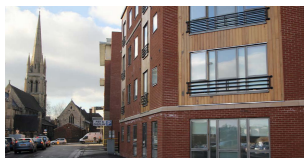
The Corner House, Lincoln
